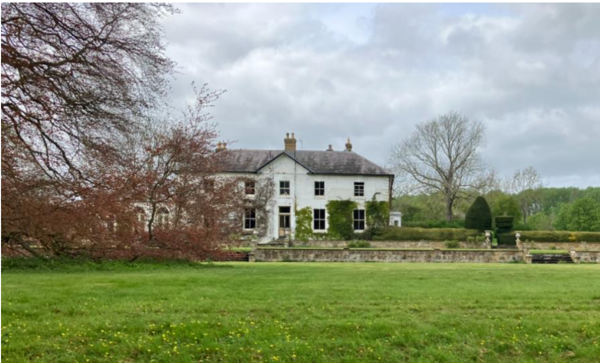
Plate 6: North east elevation of Chadshunt Hall, which looks across its own grounds towards SG13.
