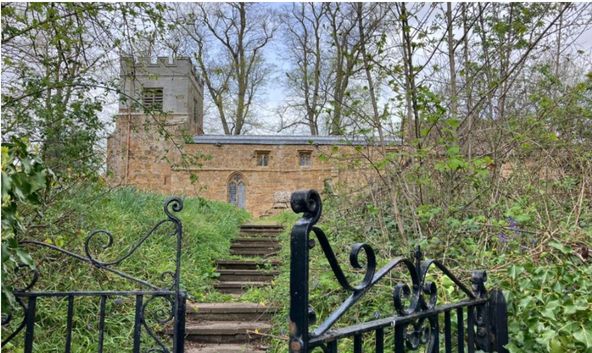
Plate 2: Footpath from Kinton Road to All Saints Church, Chadshunt, south elevation.
