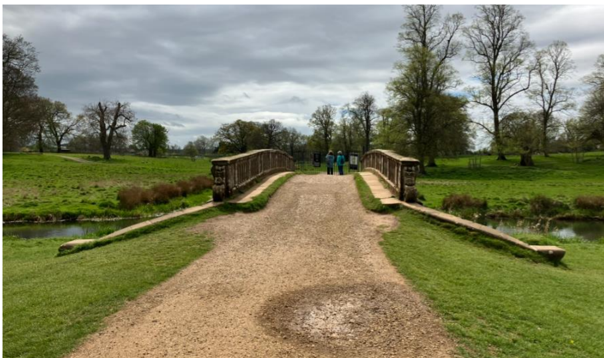
Plate 12: View south across bridge towards SG15 and SG16 to east on left
