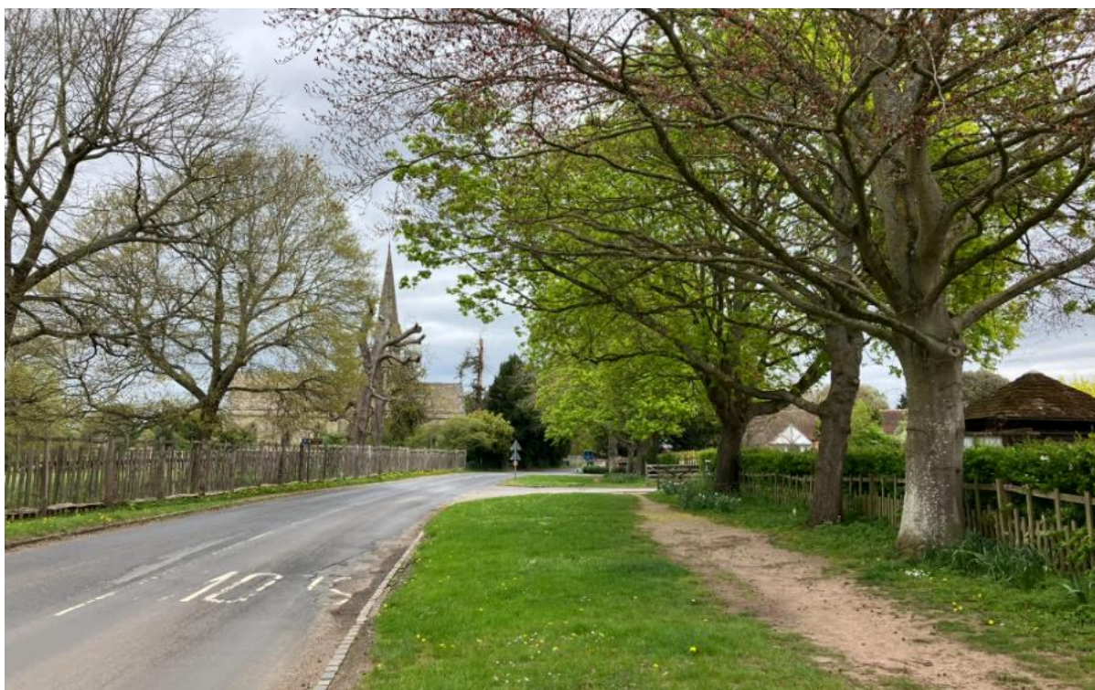
Plate 12: View north along Birmingham Road, Charlecote Park to east on left, National Trust car park and SG15 to west on right
