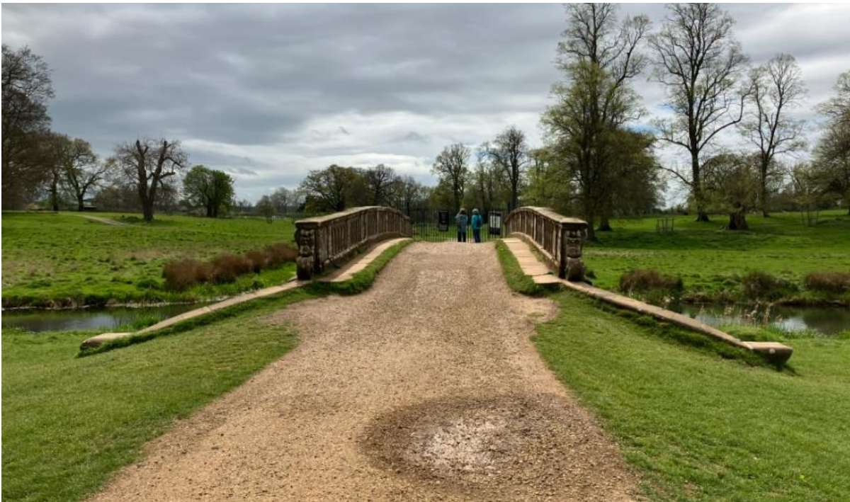
Plate 20: View south across bridge towards SG15 and SG16 to east on left
