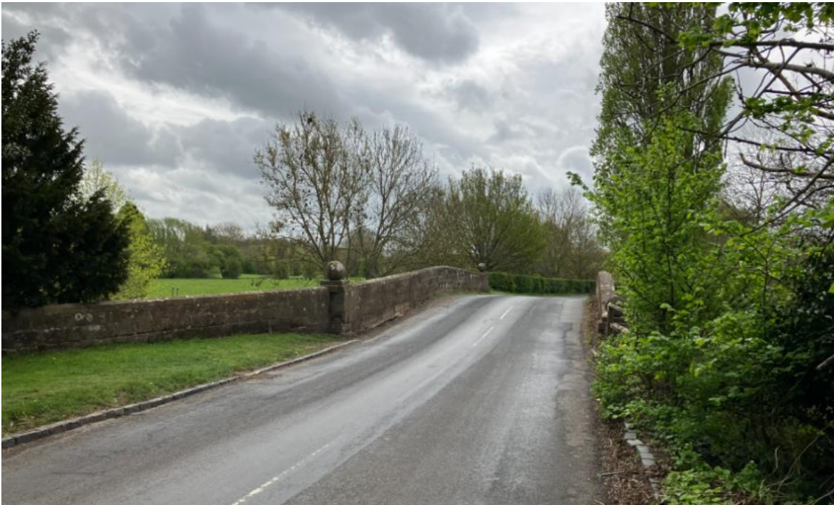
Plate 23: View looking south east across Hiorn's Bridge, Birmingham Road.
